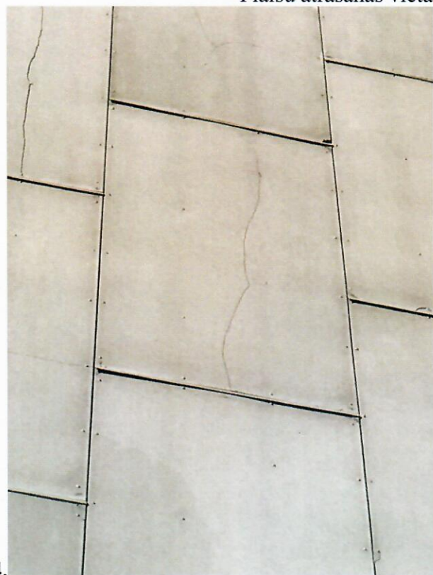
Plaisas fibrocementa loksnēs
