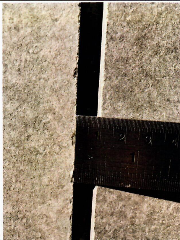
Attālums starp fibrocementa loksnēm ~9 mm
