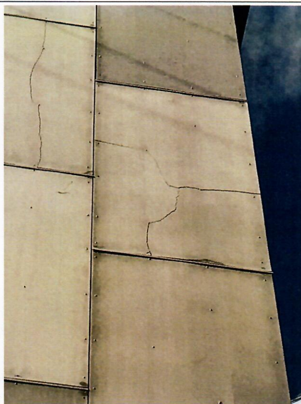
Plaisas fibrocementa loksnēs
